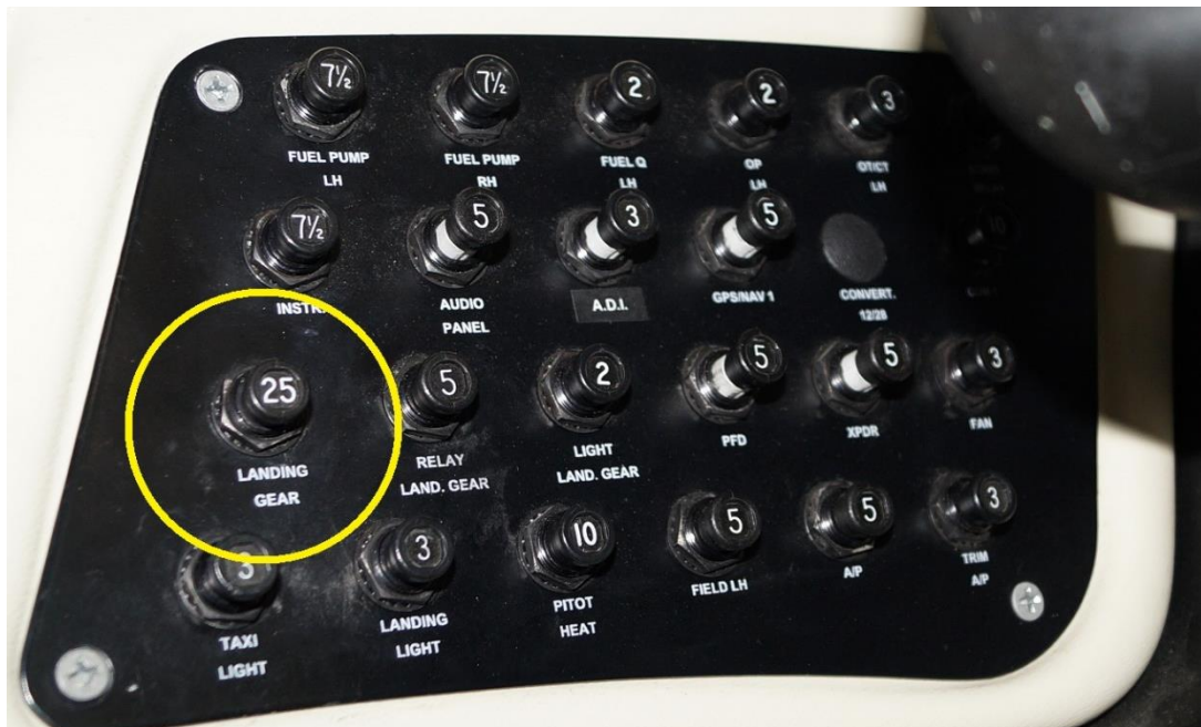
Fig. 8. The circuit breakers panel of the Tecnam P2006T aircraft with the marked "LANDING GEAR" circuit breaker
