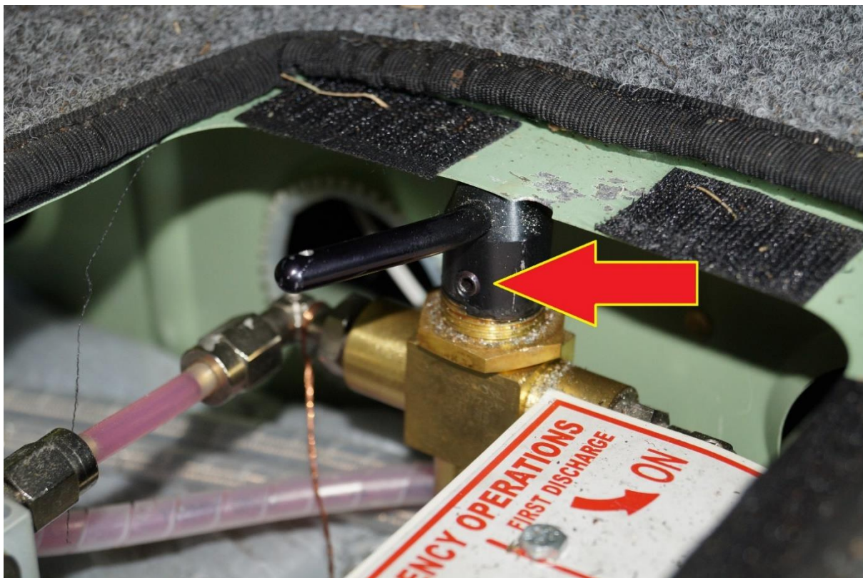
Fig. 11. Connection of the lever with the right-hand valve of the emergency landing gear extension system. The arrow marks the grub screw that prevents the free rotation of the lever on the valve shaft
