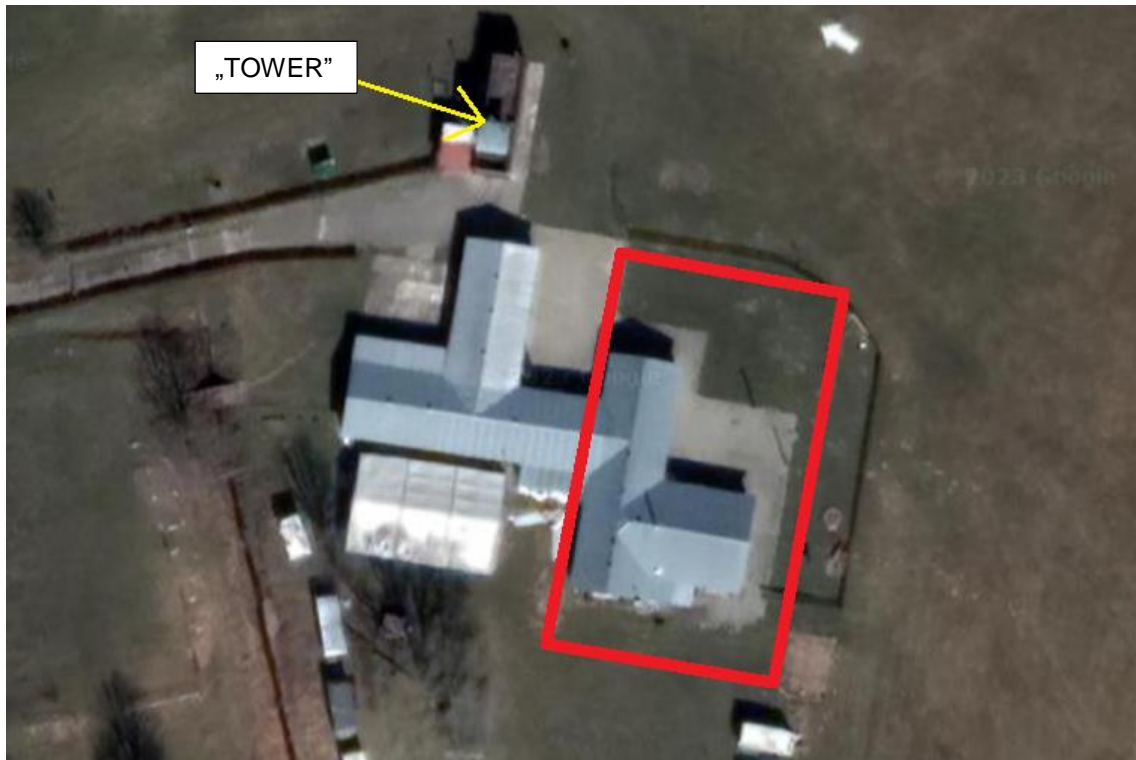
Fig. 4. The building on the airfield partially destroyed during the accident of the SP-WAW aircraft. The destroyed part of the building is marked with a red frame. [source: https://www.google.pl/maps ].
