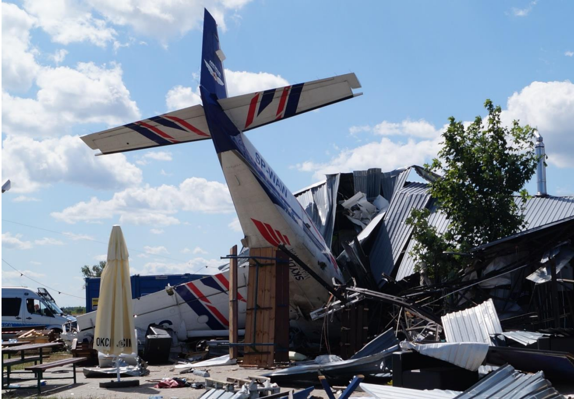
Fig. 2. Cessna 208B, SP-WAW – the wreckage before separating from the structure of the building (the photo shows a table supporting provisionally the tail of the aircraft to prevent its accidental movement).
