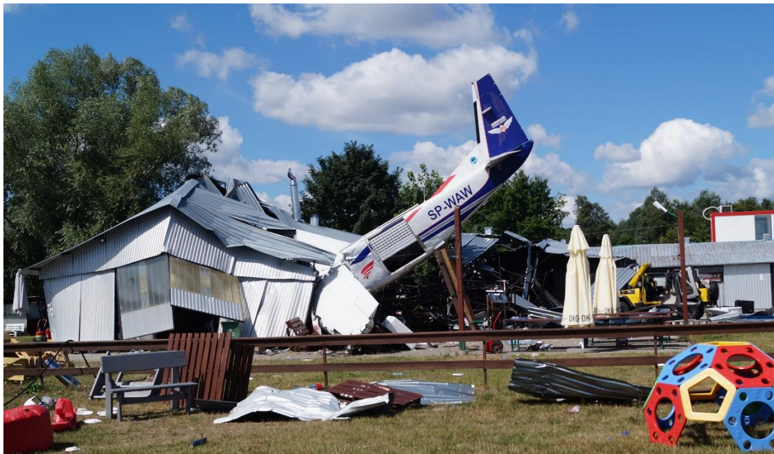
Fig. 5. Destroyed building located on the EPNC landing site. Umbrellas, benches, tables and elements of a playground for children are visible in front of the building.
