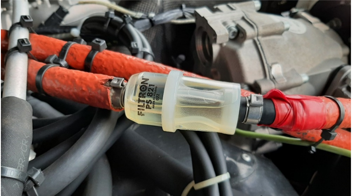
Fig. 17 Fuel in the filter on the engine [source: PKBWL]
