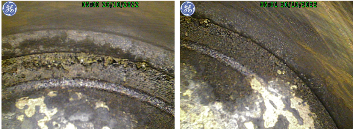
Fig. 15 Borescope camera photographs of the interior of cylinder no. 1 [source: PKBWL]
