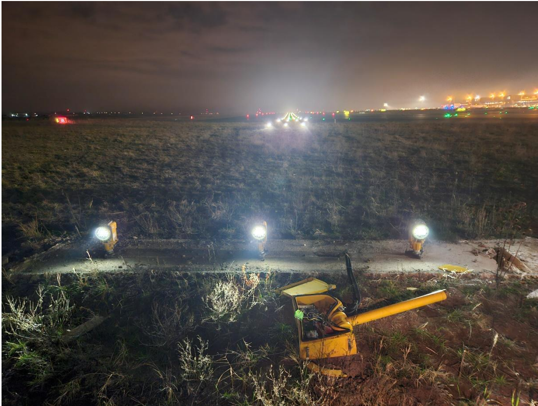
Figure 16. Damage to the lighting system – second row of lights from the end of the runway
