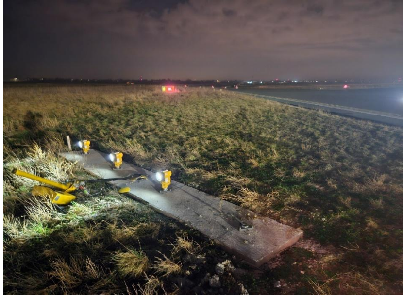
Figure 17. Damage to the lighting system - first row of lights approximately 150 meters from the runway threshold
