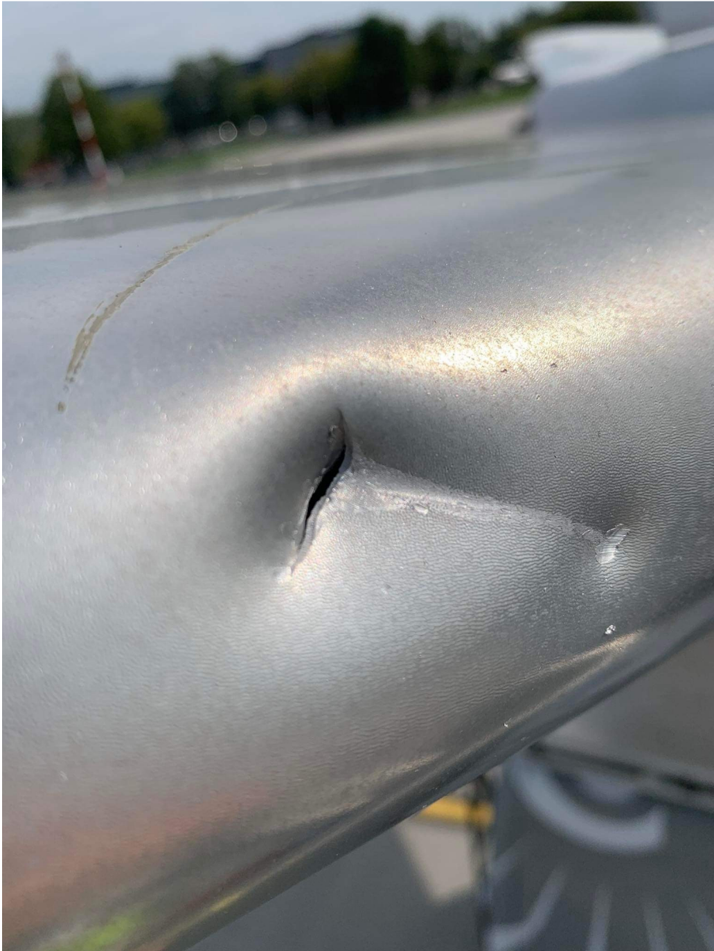
Fig. 6. Dent and crack on of leading edge on leading edge of the right side horizontal stabilizer.
